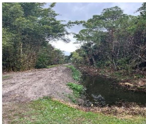
Figure 10. Canal Bank Clearing on Canal 6
