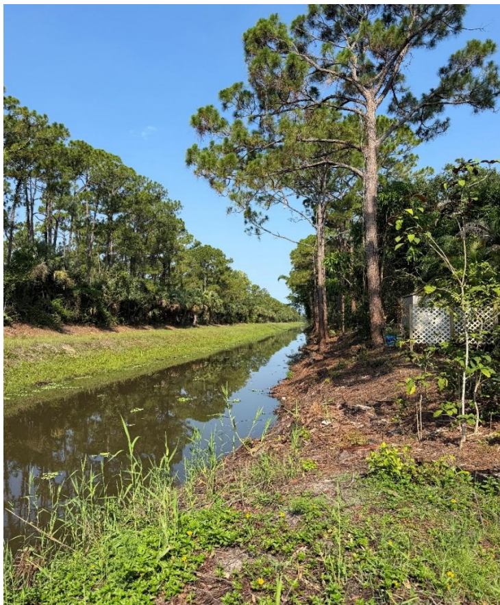
Figure 7. Completed Phase 2 Hurricane Milton Storm Debris Removal
